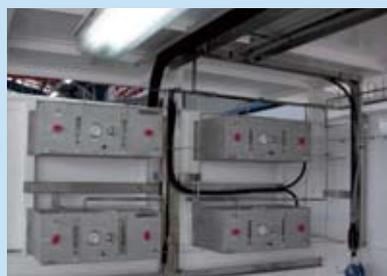
Sample Conditioning Systems (SCS) for natural gas. The SCS is installed close to the sampling point and reduces pressure from process conditions to 1-2 bar. The method of construction assures that the mercury concentration in the sample stream remains unaltered when flowing through the SCS.
