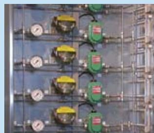
Sample point multiplexer unit. Up to 16 sample streams can be connected to the multiplexer inlet. For minimum response times, the sample lines are continuously purged to keep them conditioned. Specially coated bypass filters retain entrained liquids (coalescing filters can also be used).
